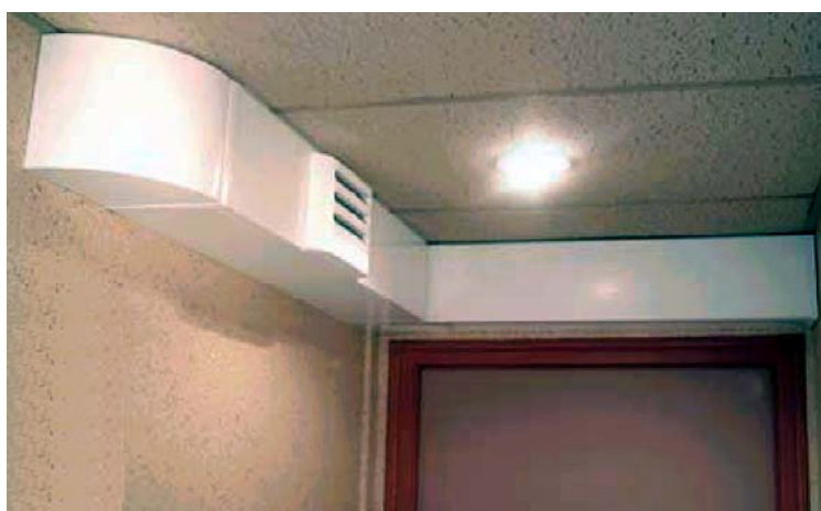
Figure 22 T2a Very Low Pressure Drop duct
